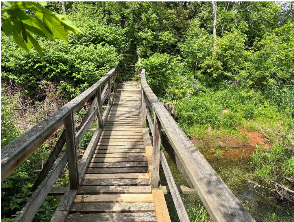
Trail Bridge at Stocking Hill Creek
